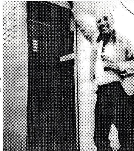
Bob supports repeater cabinet.
