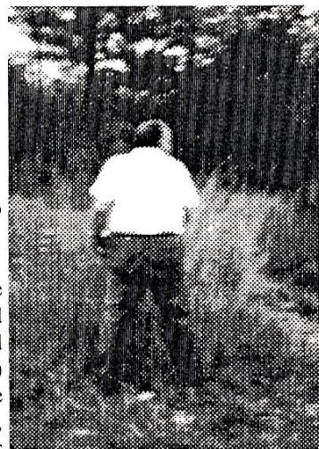
Herb improves tower ground connection.
